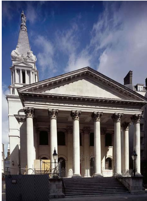
Façade of St George's, post-restoration Image from WMF website http://www.wmf.org.uk/projects/view/
