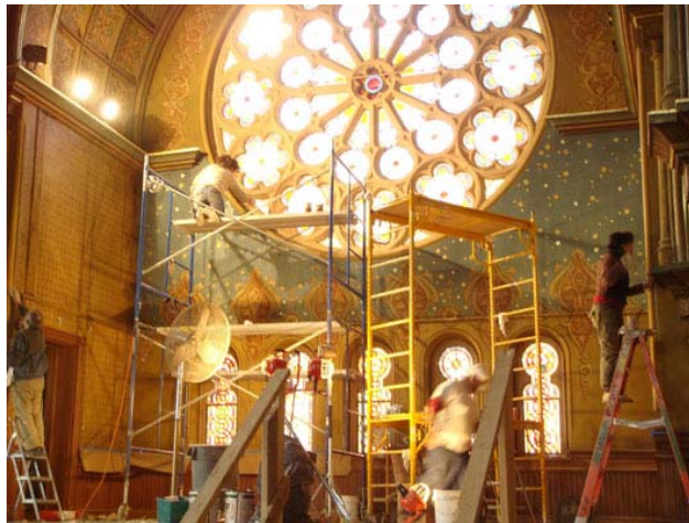
Restoring paint on the balcony, photo Evergreene Painting Studios.
