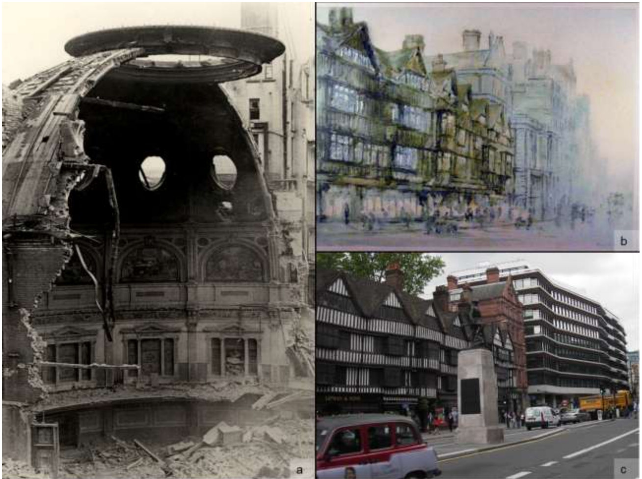
Figure ix. (a) The central banking hall and great dome of the Birkbeck Bank revealed during its demolition in 1962, from N.Taylor, 'Ceramic Extravagance' Architectural Review 138, 825 (1965): 320 © Architectural Review and reproduced by kind permission of Architectural Review. (b) its Holborn frontage shortly after completion c. 1903 © Birkbeck, University of London and reproduced by kind permission of Birkbeck College. (c) its replacement, the National Westminster building in 2013. The NatWest building is constructed to the same footprint as its predecessor and the floor plan is remarkably similar.
