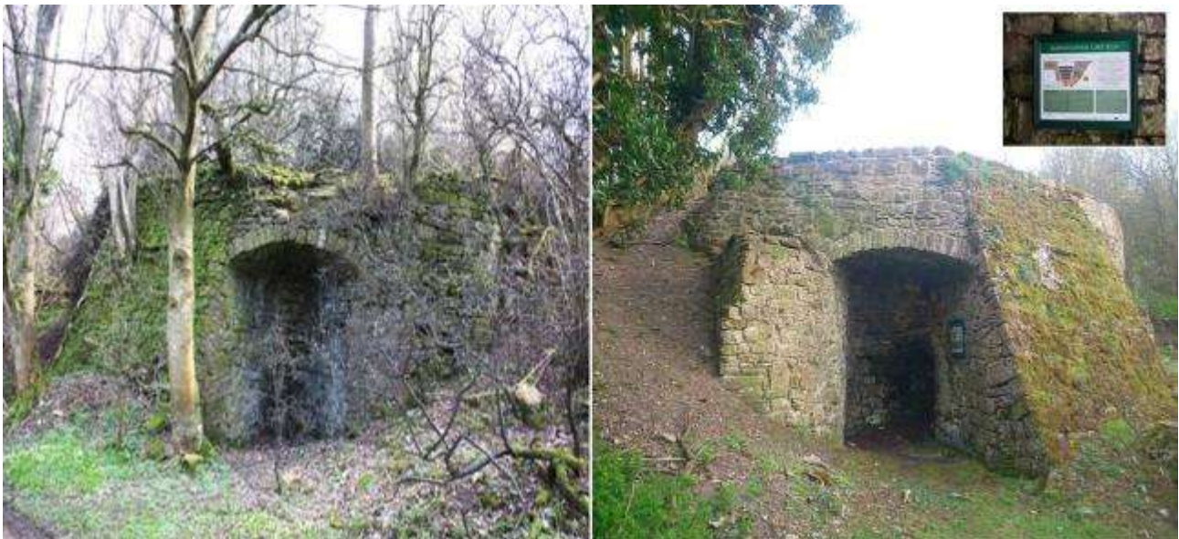
Figure 12 Barningham Lime Kiln (one of the CIF projects) before (left) and after stabilisation and removal of encroaching scrub (right) with (inset) interpretive plaque
