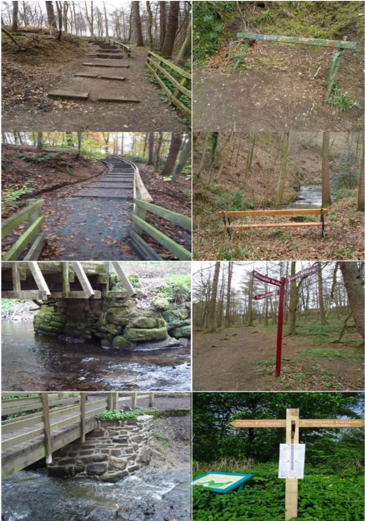
Figure 21 Old and new; access improvements - reinstated footpaths, benches, bridges and signage in Flatts Wood
