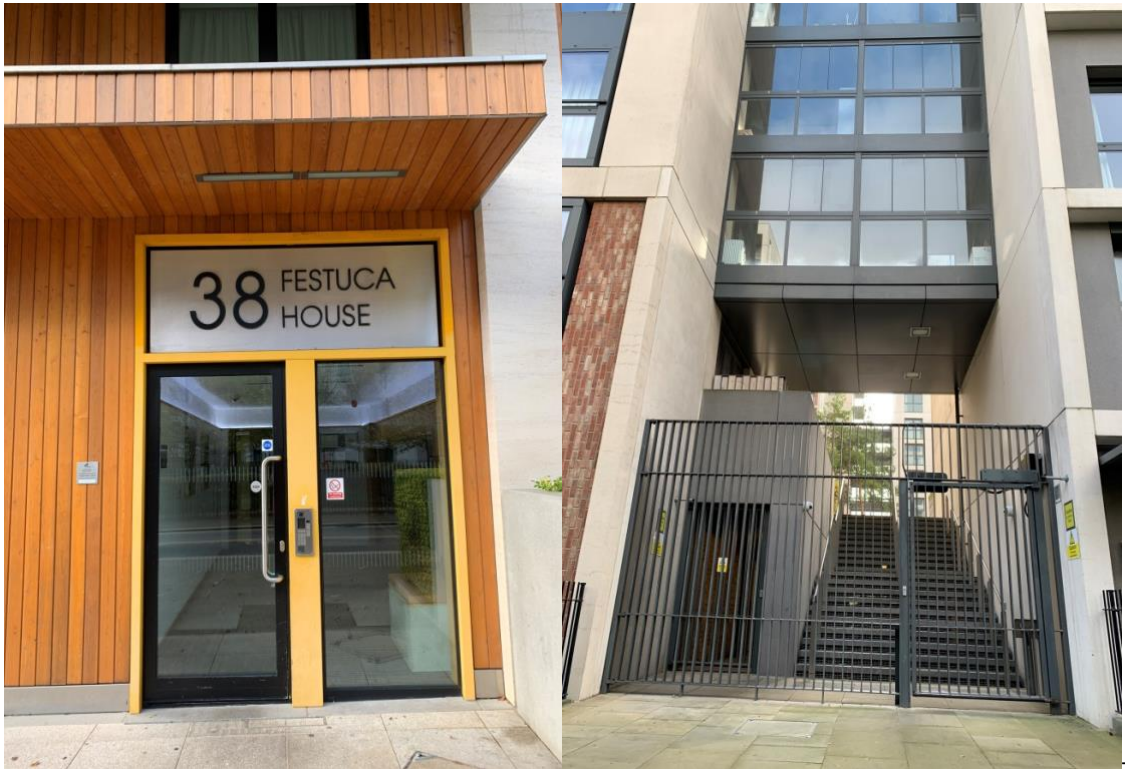
Figure 3: East Village's Secured Doors and Gates
