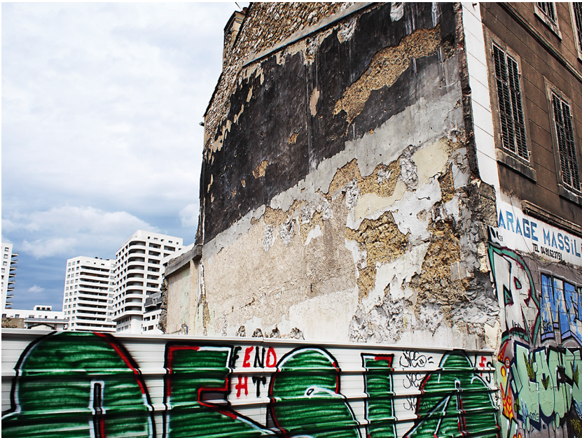
Image 5.3: Demolition and reconstruction, north Boulevard National.
