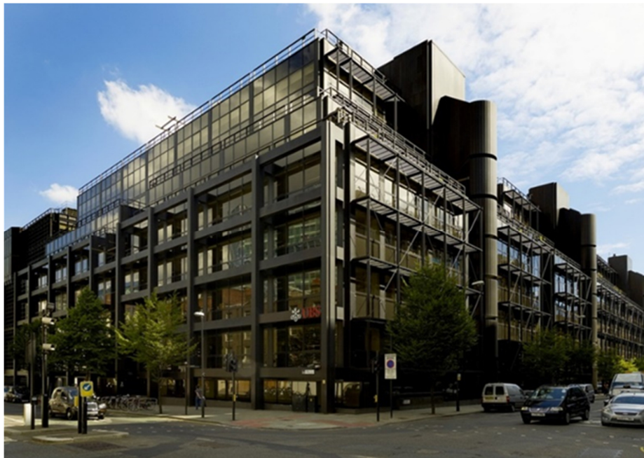
5.5 Arup Associates: Numbers 1-3 Finsbury Avenue, 1982-1985. (Source: Ken Powell, Arup Associates , Swindon: Historic England, 2018.)
