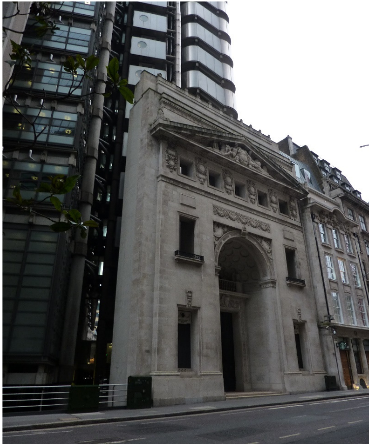
3.6 Lloyd's building, retained portal from the Cooper building. (Source: author's photograph.)
