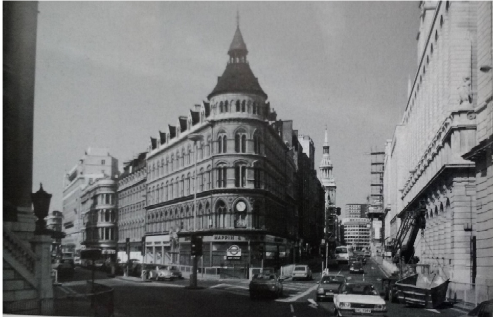
2.2 Mansion House site from Bank Junction, c.1984. (Source: Gavin Stamp, Lost Victorian Britain , London: Aurum, 2010.)
