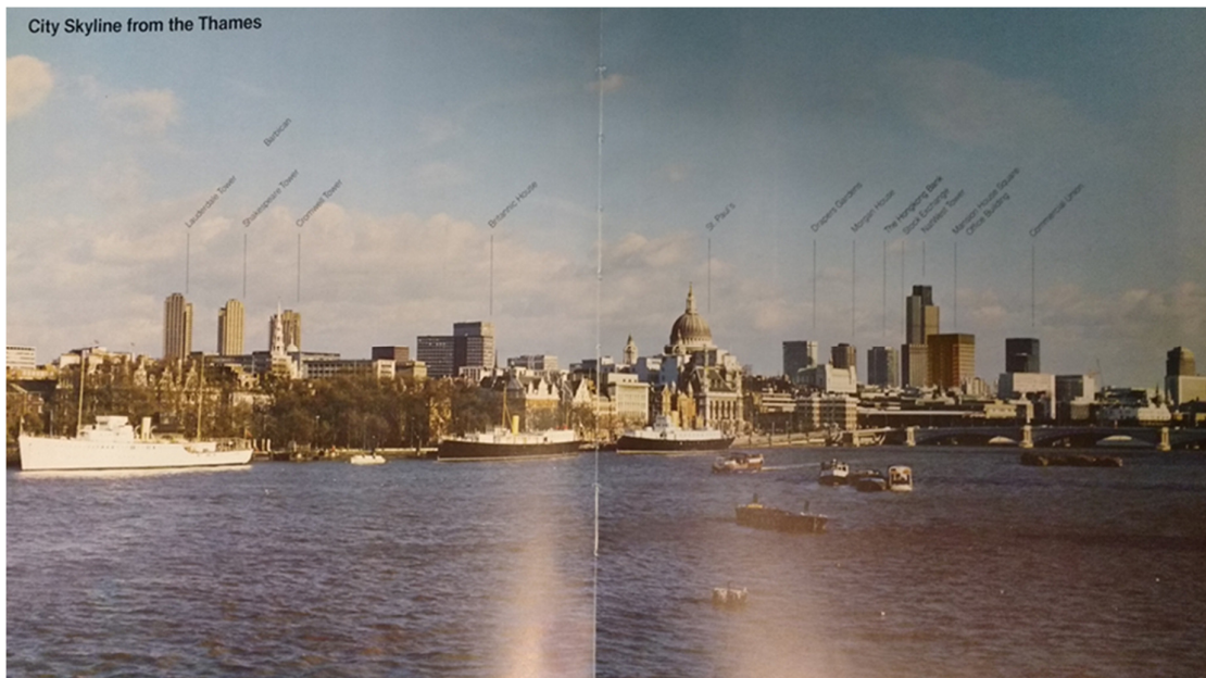
1.6 City skyline, c.1980. This illustration appeared in the Peter Palumbo's promotional book, The Mansion House Square Scheme (London: Number 1 Poultry Limited, 1981), to demonstrate the impact of the proposed Mies van der Rohe tower, an image of which was inserted.
