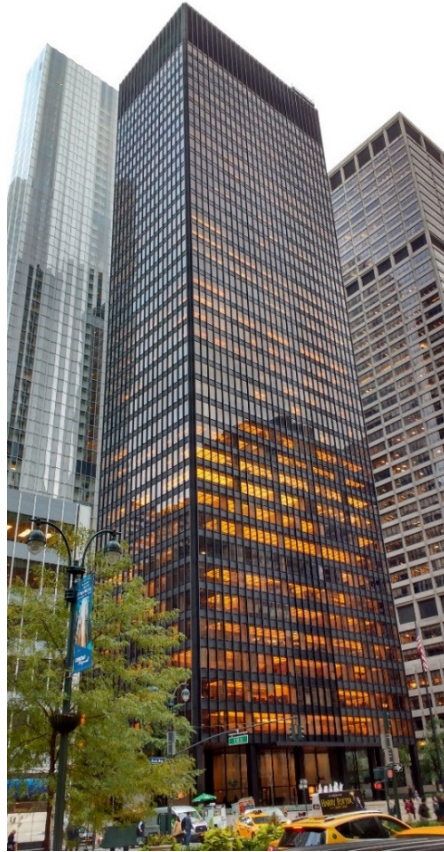
2.4 Mies van der Rohe: Seagram Building, 1954-1958. (Source: author's photograph.)
