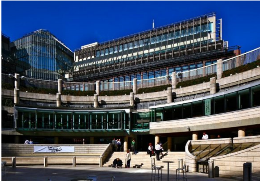
5.13 Broadgate Circle following completion of the UBS building. (Source: Twentieth Century Society.)
