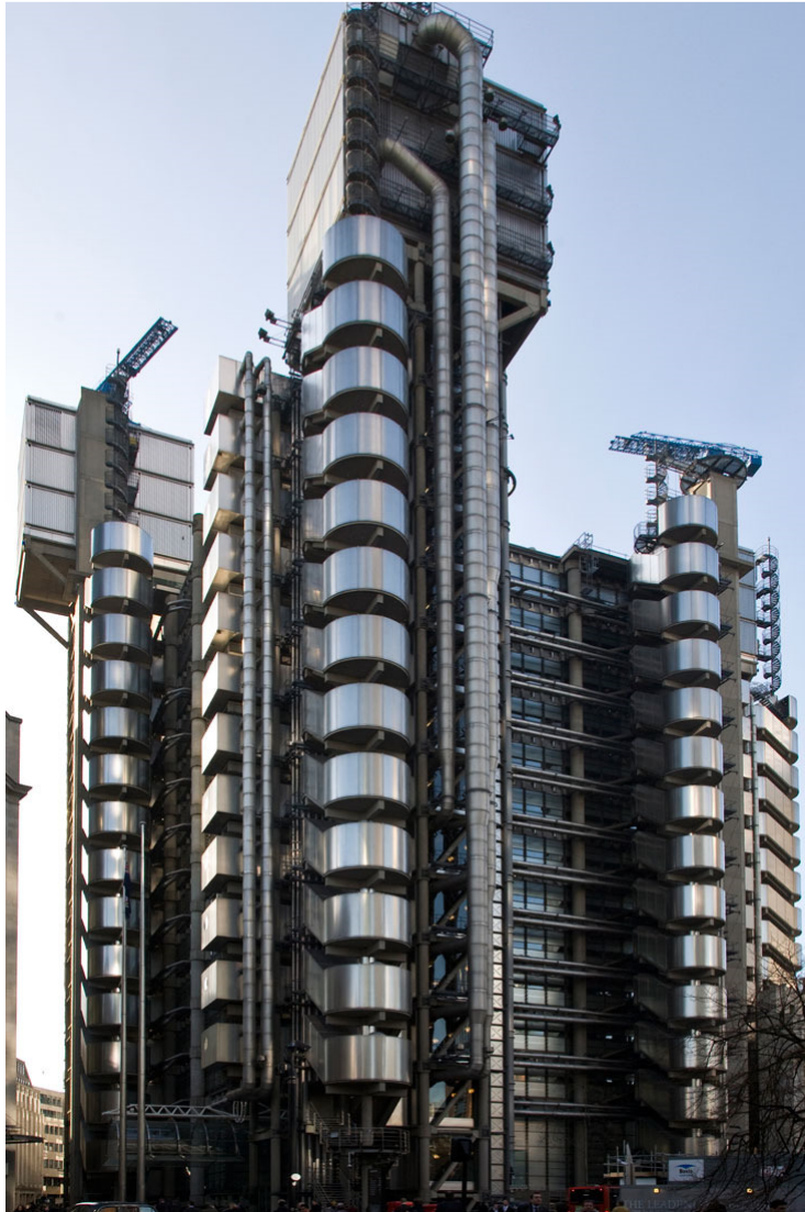
3.3 Richard Rogers Partnership: Lloyd's building, 1981-1986. (Source: Lloyd's of London website.)
