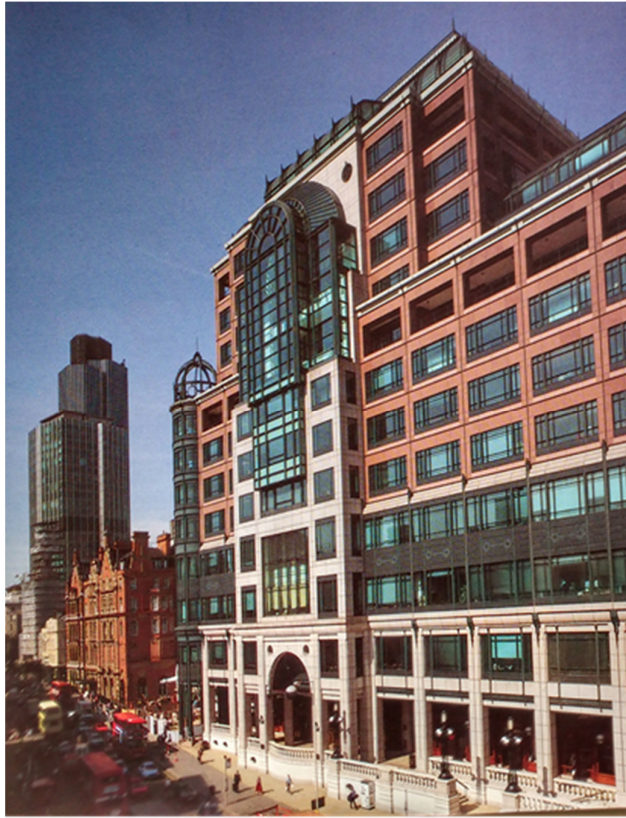
5.7 Skidmore, Owings and Merrill: Broadgate, Bishopsgate frontage. (Source: Broadgate and Liverpool Street Station , London: Rosehaugh Stanhope Developments, 1991.)
