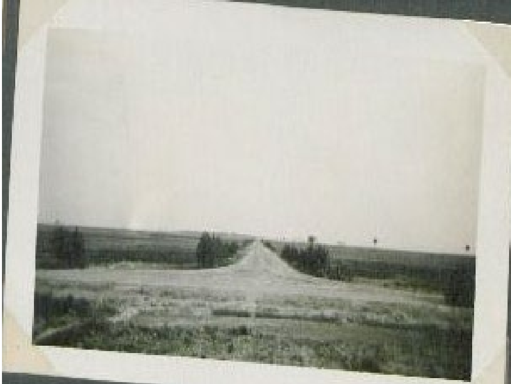
Detail of Image 33 showing photograph 25
