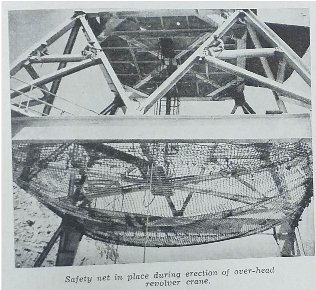
Image 46: Anon., 'Safety net in place during erection of over-head revolver crane', photograph, Commemorative Volume , BBMB, Chandigarh.
