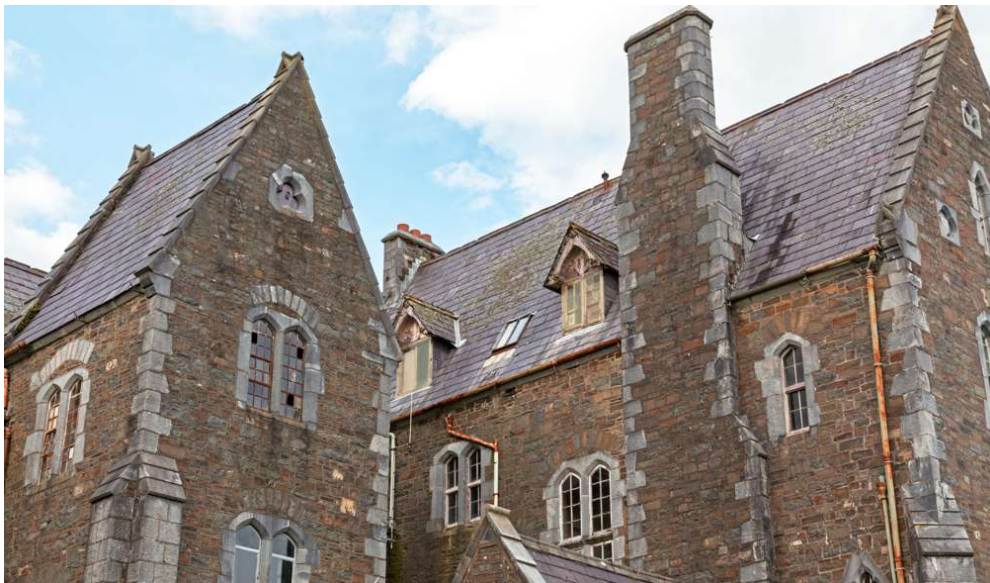
Figure 2.9 Killarney: Cut stone detailing.
