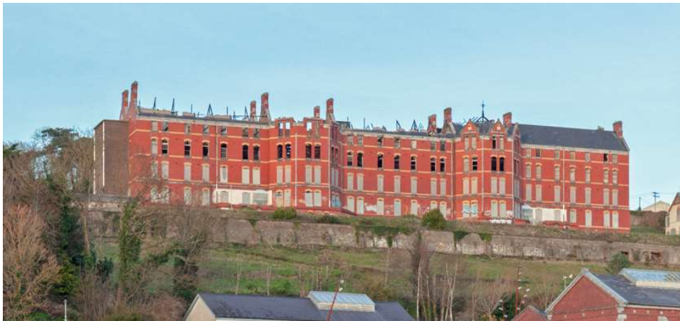
Figure 3.8 Cork: Auxiliary ward block, William Hill, opened 1894.
