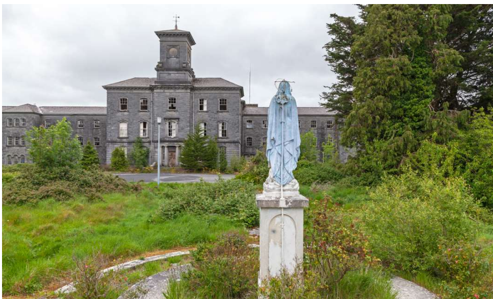
Figure 5.13 Ennis: Unsecured and deteriorating.
