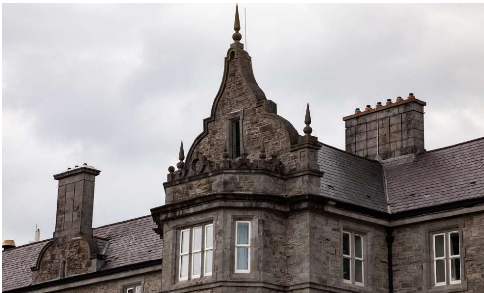
Figure 2.12 Sligo: Cut stone detailing.
