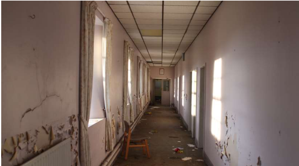
Figure 5.15 Ballinasloe: Internal modernisation, c.1970s-80s.
