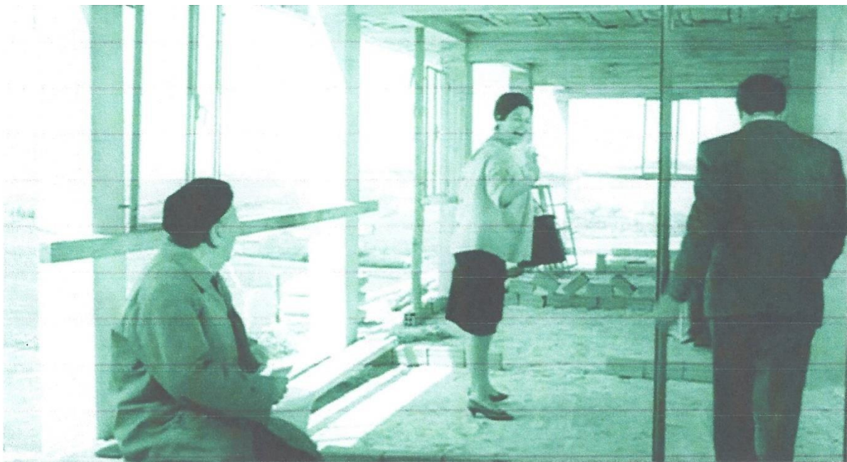
Fig. 20: El verdugo : the new flat under construction (minute 39).
