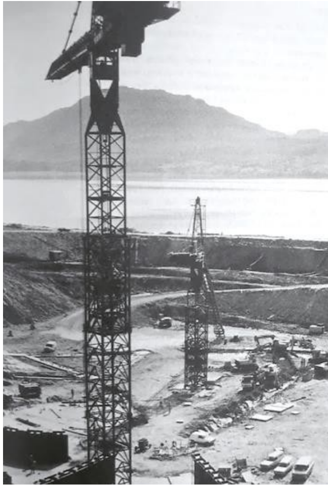
Fig.63 'Loch Kishorn construction site' Caption for Untitled Fay Godwin, Photograph, 1975
