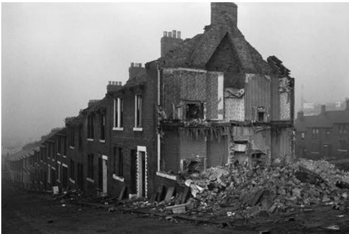
Fig.56 Demolition, 1971 in Byker, 1983 p.120. Photograph, Sirkka-Liisa Konttinen 1971
