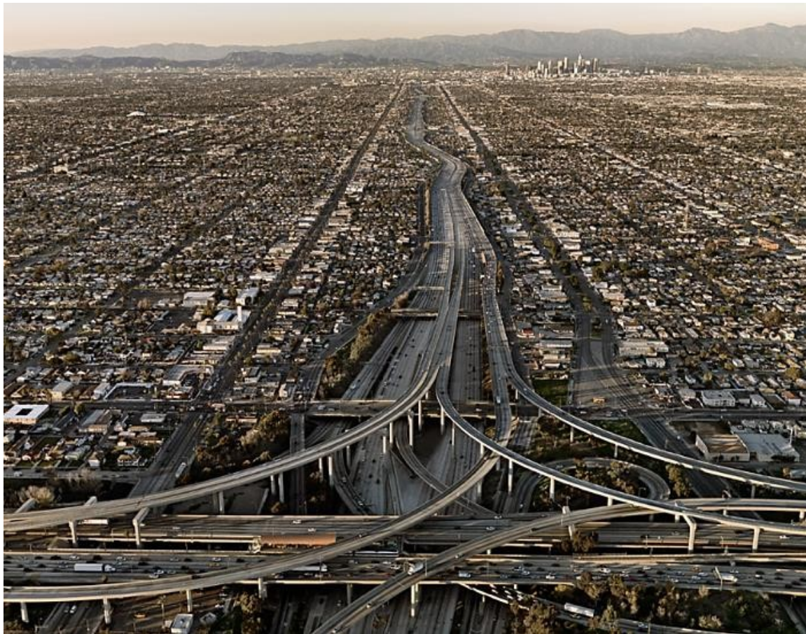
Fig.72 Highway # 5 Los Angeles, California, USA
